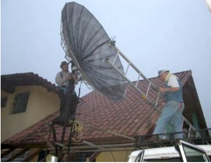
Figure CsLD 5: Carlo and Ermanno disassembling the satellite dish supplied by Mr. Ismael Santos.
