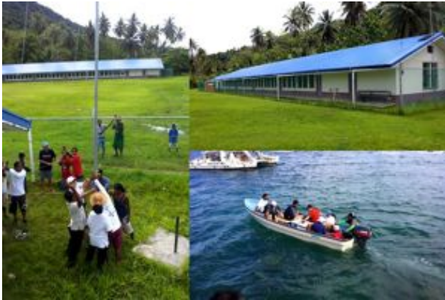
Figure CSP 4 : Mounting the pole mast in Udot
