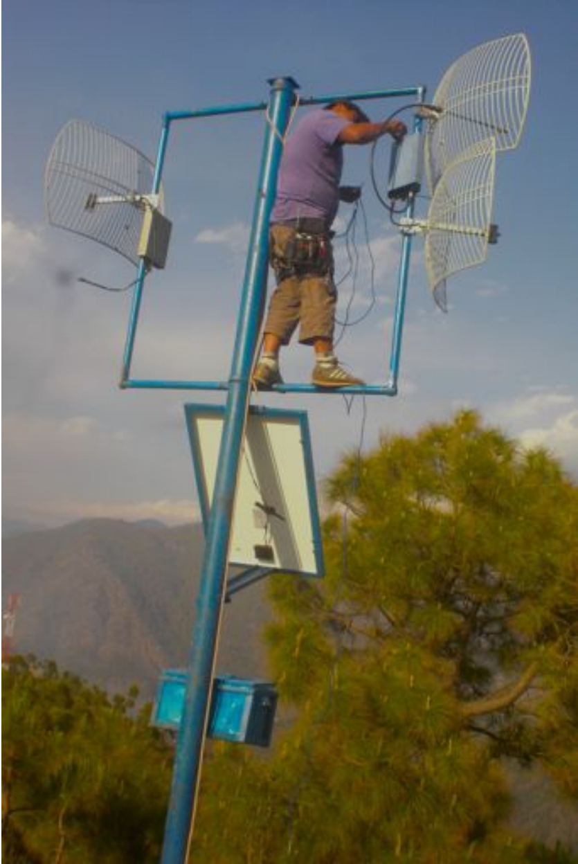
Figure CSD 8: Backhaul Relay, Garhwal Network
